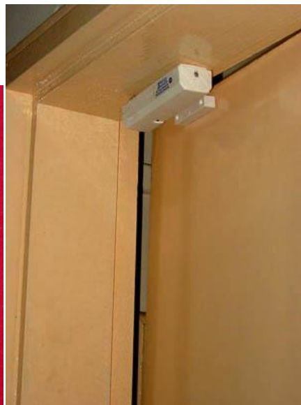
Figure o: Different types of door status sensors (only ever used as part of a CBL07 controller)
